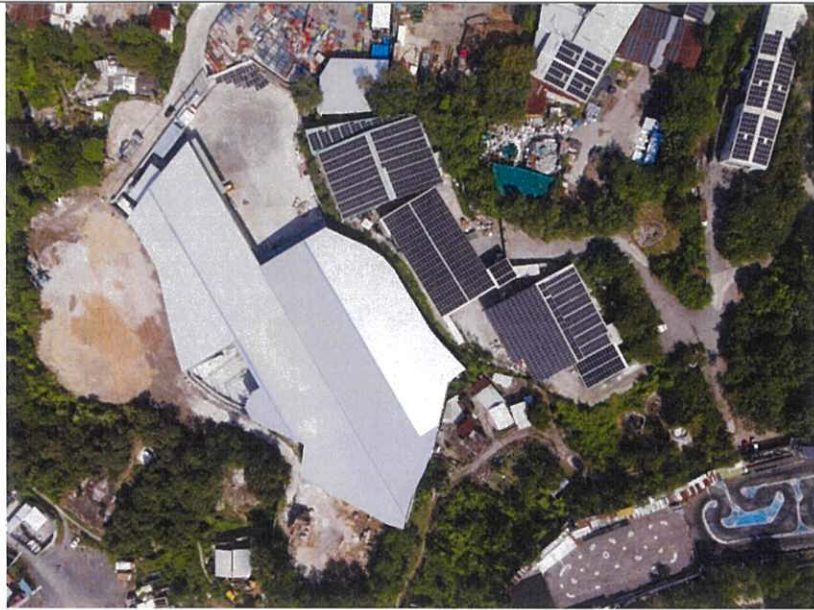
Aerial Photo: Overview of the Site
