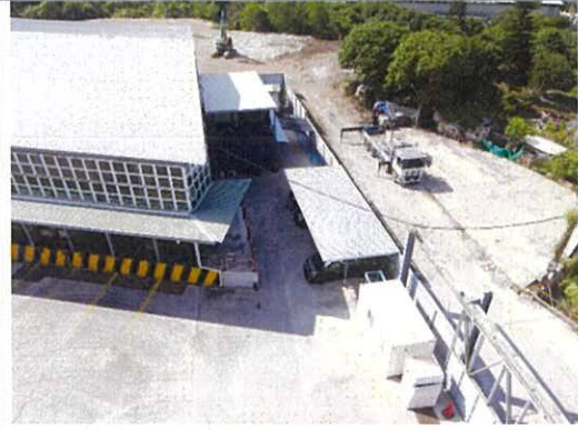
Aerial Photo 6: Site Entrance
