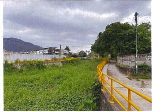
Site Photo 2: Final Discharge to Wong Tong Stream ( Maintained by DSD)
