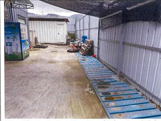
Site Photo 4: Existing 1m (W) x 1m (H) in the site
