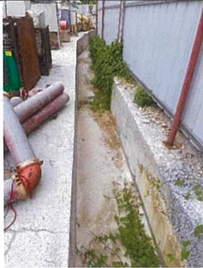
Site Photo 3: Existing 1m (W) x 1m (H) in the site
